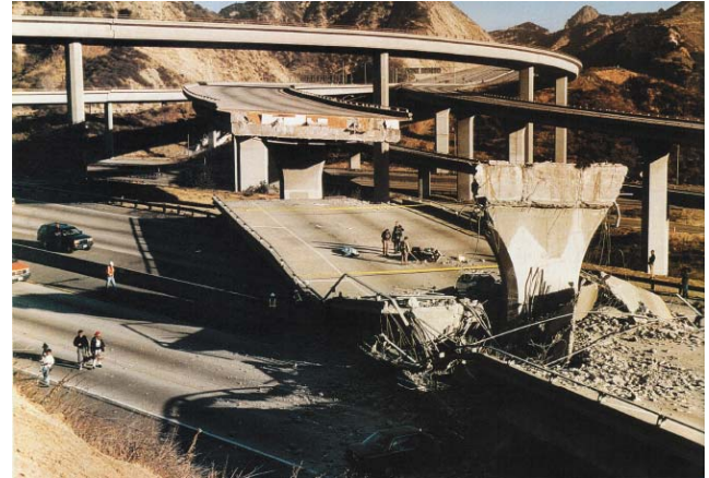
Collapse of portion of the I-5 Freeway following the 1994 Northridge Earthquake
