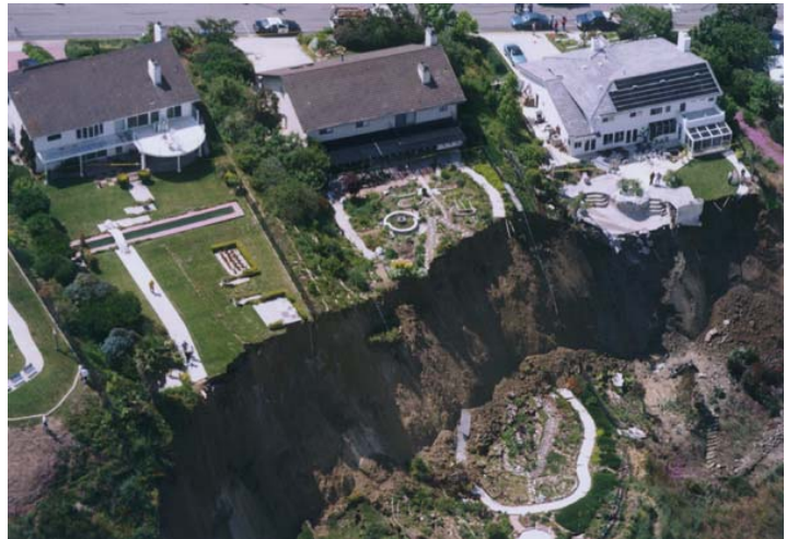
Landslide failure in Laguna Niguel
