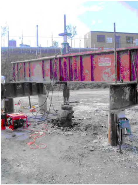
Figure 7. Load testing frame for testing under axial tension.
