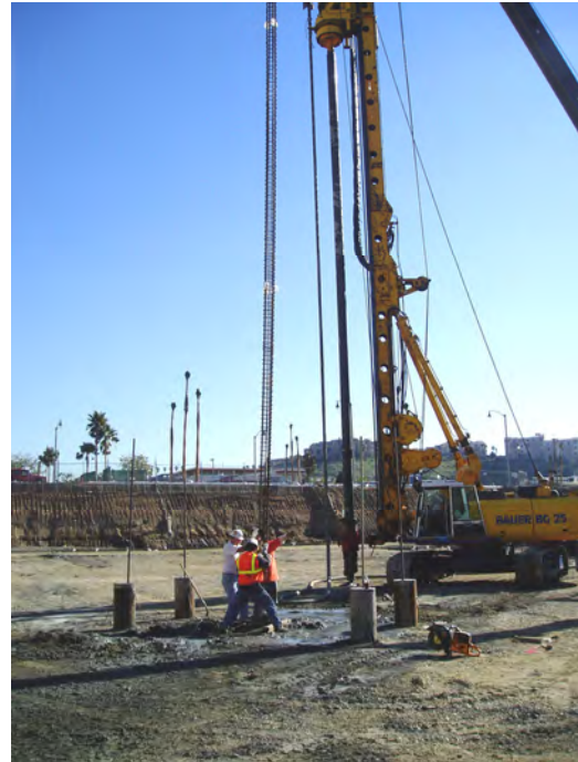
Figure 4. Installation of APGD pile by Wet Dip Method. Note “Wet Dipping” of rebar cage into grouted pile.
