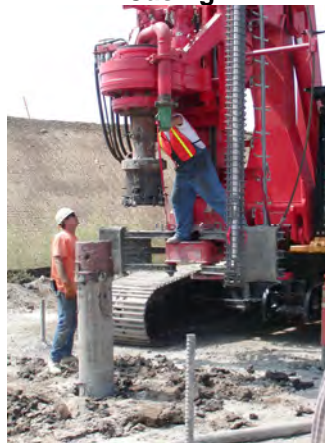
Drill head detached from Casing
