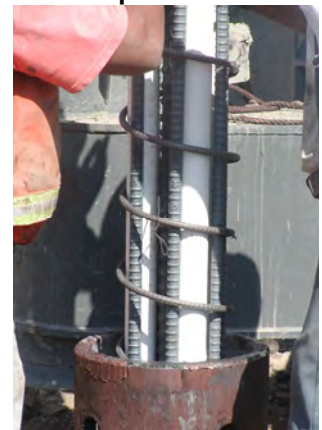
Inserting Rebar Cage with Inspection Tubes
