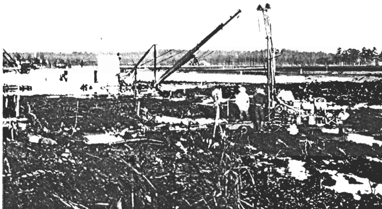
FIGURE 8 - DREDGE IN OPERATION
