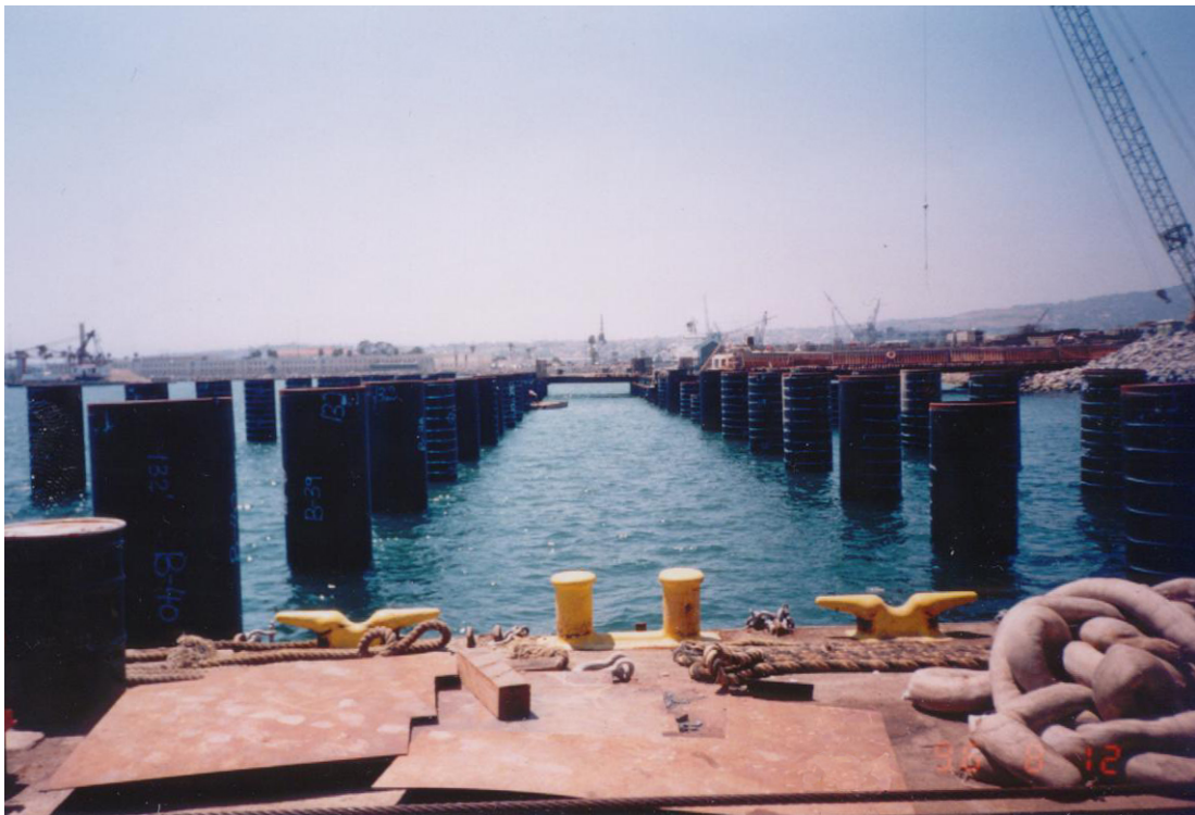
Pipe Pile Supports for LAXT Wharf
