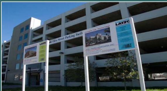
Los Angeles Community College Parking Structure
