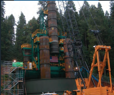
Middle Fork Surge Shaft
