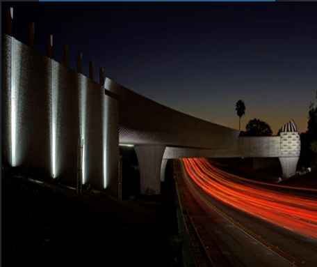
I-210 Iconic Bridge
